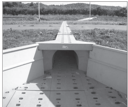
Wildlife can use the purpose-built passages beneath roads
